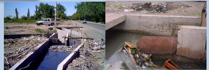
Figure 3: Urban waste in irrigation canals: reduced distribution and application efficiency
